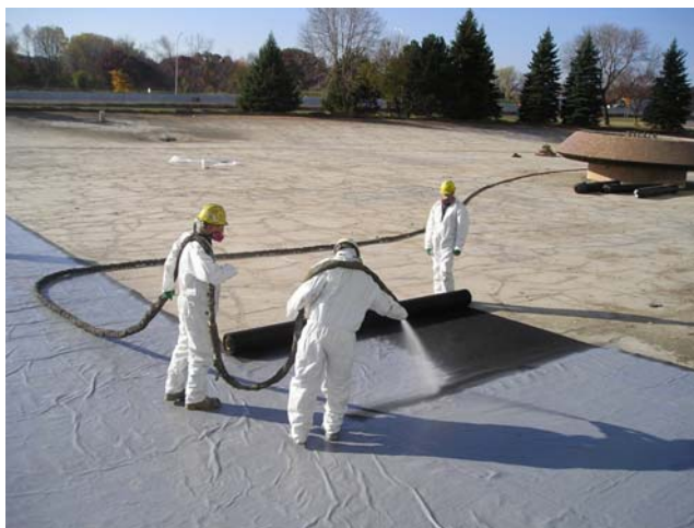
Figure 1: Installation of a polyurea geomembrane.
